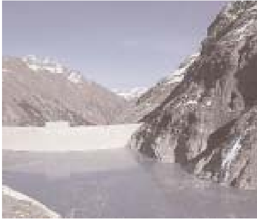
Measurement and evaluation of the protection to lightning of a dam
